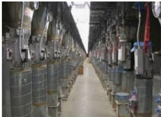
Figure 85 – State-of-the-Art White Oak Infrastructure: Advanced Air Terminal Units Supporting Laboratories
